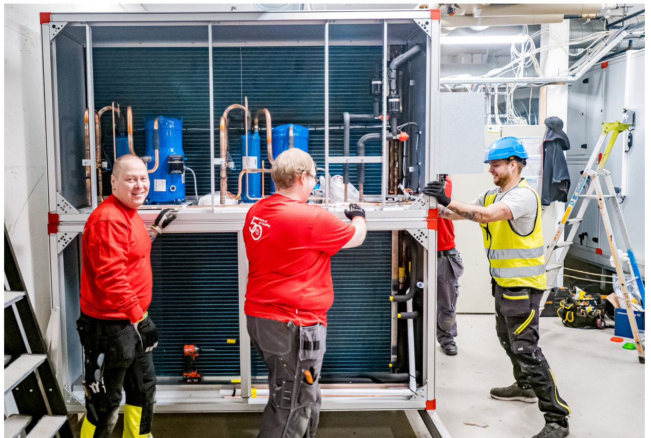
The splittable, integrated reversible heat pump ThermoCooler HP is placed into position.
