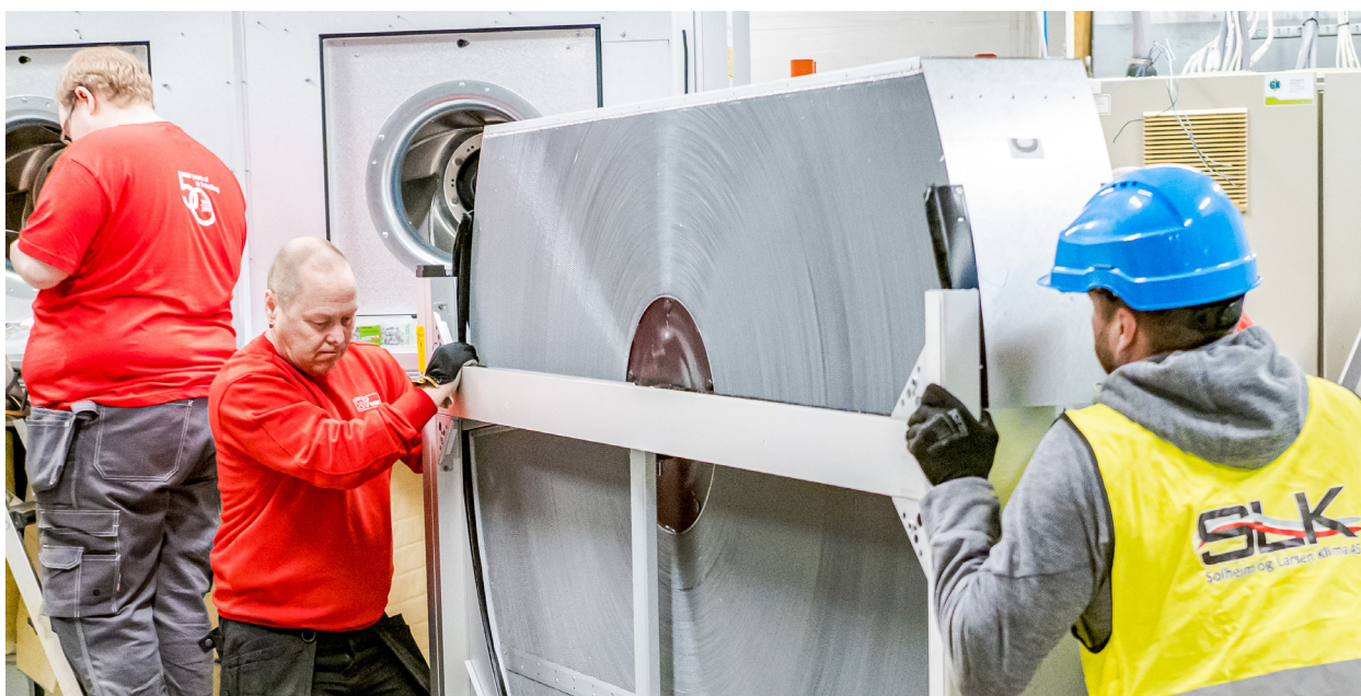
Employees from IV Produkt and Solheim og Larsen Klima AS cooperate to put the split thermal wheel in place.
