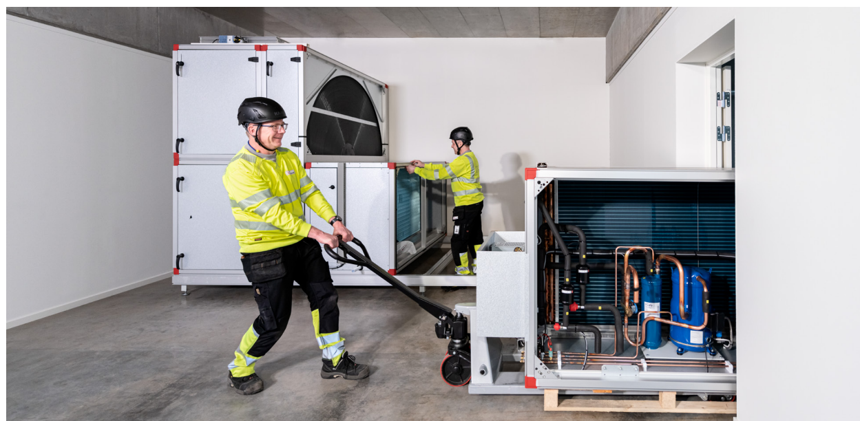
Pär and Ola from IV Produkt transport a size 600 Envistar Flex AHU with integrated reversible heat pump ThermoCooler HP through a standard door.
