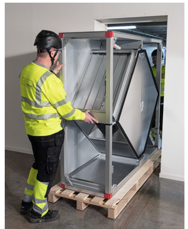
The split counter-flow heat exchanger is transported through a 90 cm wide door opening.
